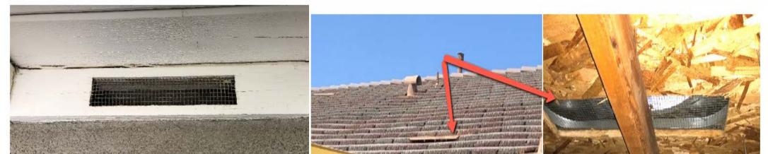
EPC/CERT is compiling inexpensive ways to install 1/8 inch screen on intake and gable vents and a list of vendors to do the work
